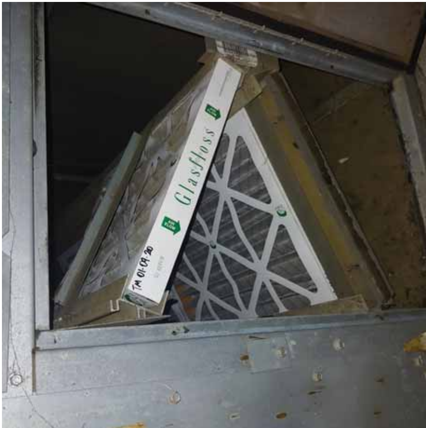
Server/PIC-ahu 2a old filters.jpg
