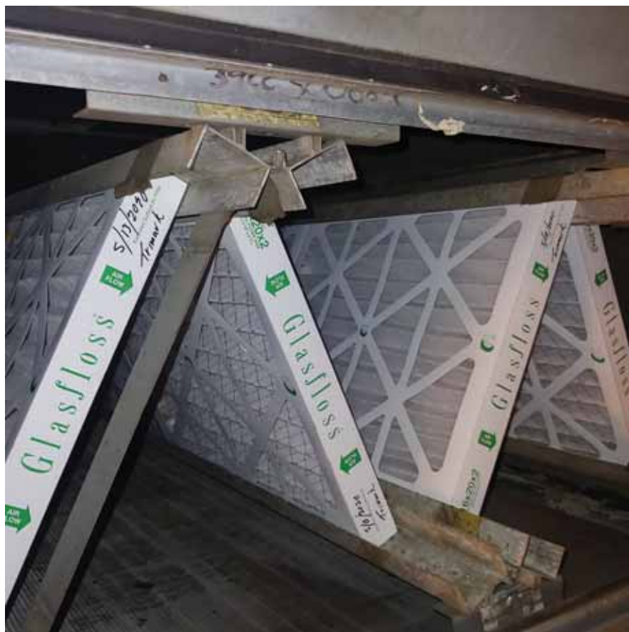
Server/PIC-ahu 5b new filters.jpg
