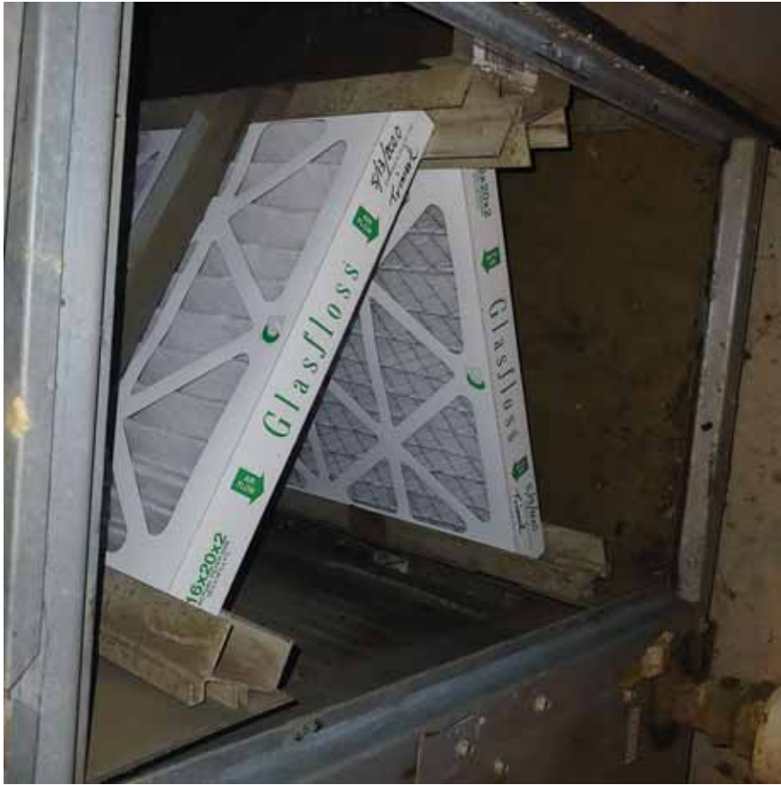
Server/PIC-ahu 2a old filters.jpg
