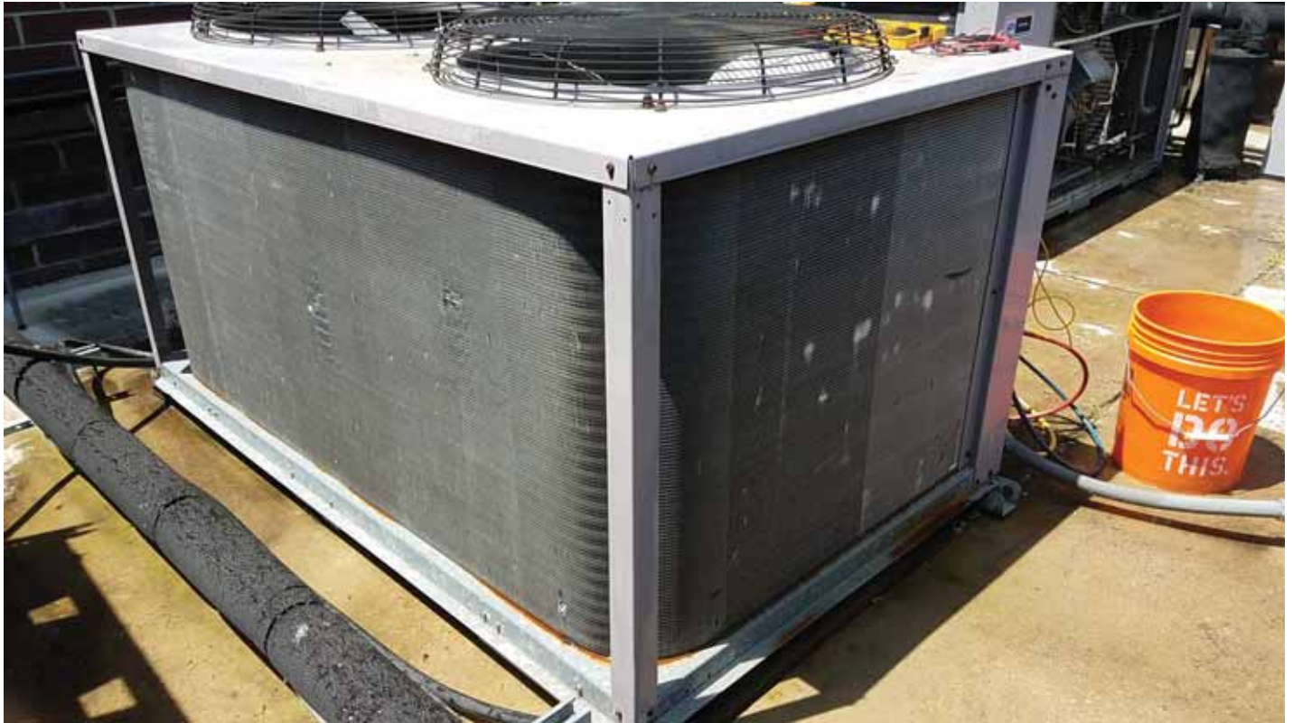
Server/PIC-CU2BCleanedCoil.jpg
